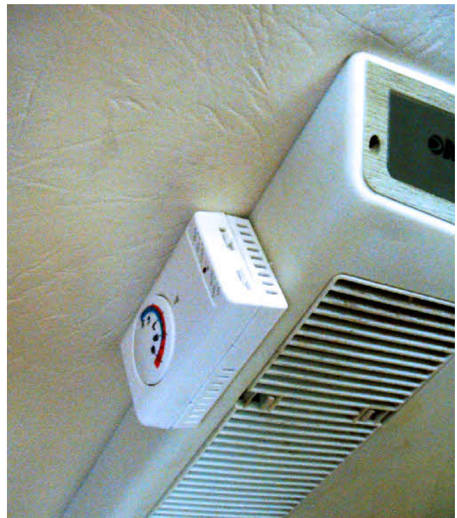
The final Installation
